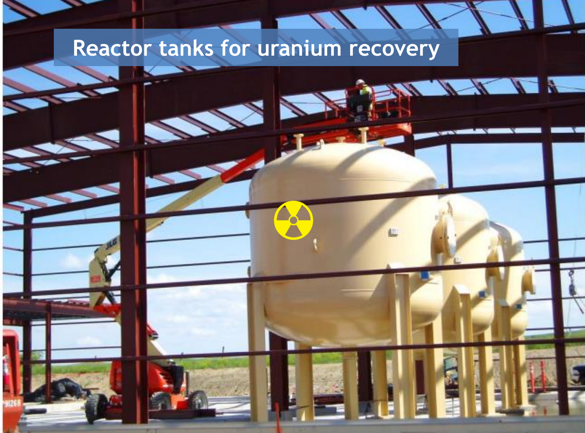
Figure 2.1.5. Reactor tanks for uranium recovery within the GPR.
